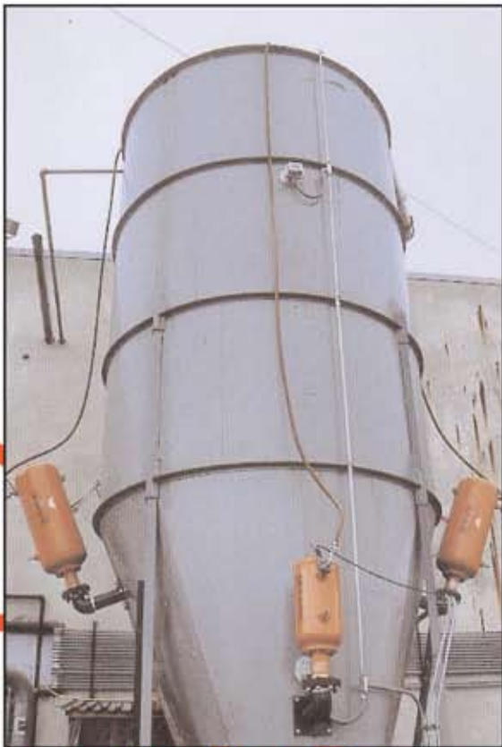
CO-GENERATION PLANT: Use ABS-4-5 blasters to feed cut-up paper bags to furnace. Ask for Bulletin 9065.
